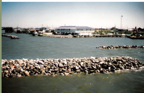
Breakwater System – Town of Grand Isle, Louisiana
