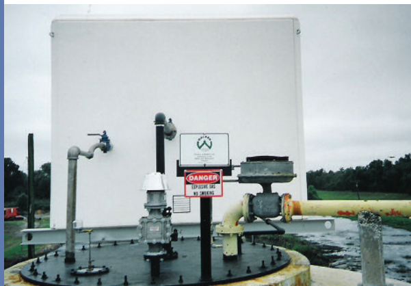
Wastewater Treatment Plant – City of Westwego, Louisiana
