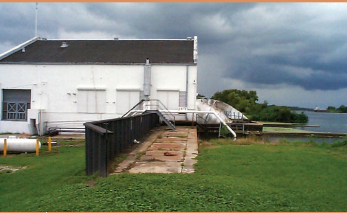
Drainage Pump Station – Belle Chasse, Louisiana
