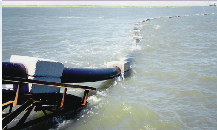
New Water Line – Town of Grand Isle, Louisiana
