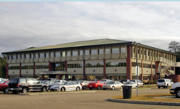
Parish Government Facility – St. Tammany Parish, Louisiana
