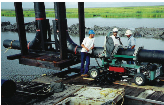
New Water Line – Town of Grand Isle, Louisiana
